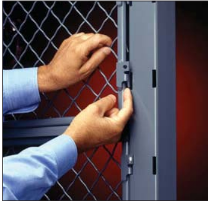
STEP 1: ALIGN HOOKS AND INSERT INTO SLOTS
